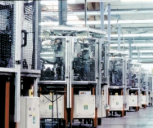
Production hall with modular automatic round table machines
